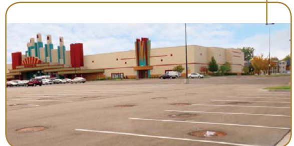
The treatment device is located underground so that the surface can still be used as a parking lot.
