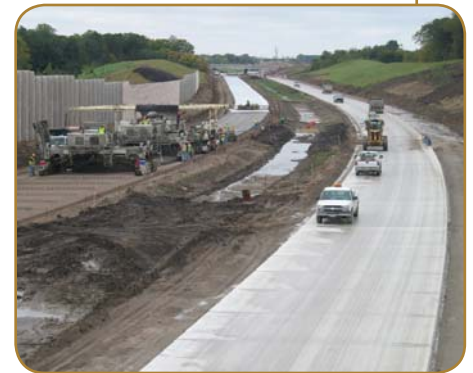
Over 10.5 million cubic yards were excavated for the project.
